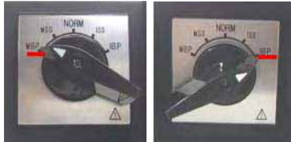
Figure 28 MBS position when installing or removing the STS module
